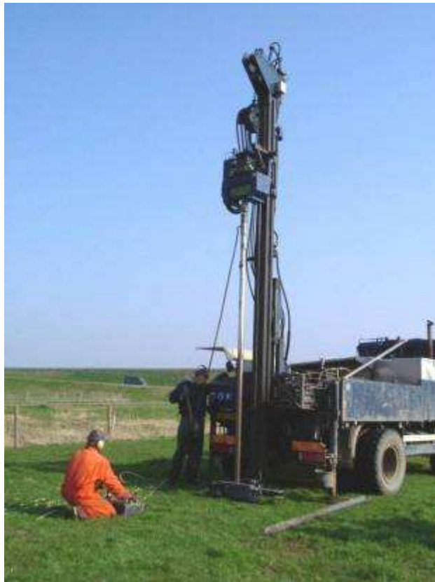
Drilling with aqua-lock
