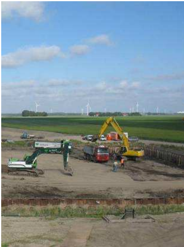
Removing 20.000 m 3 top soil
